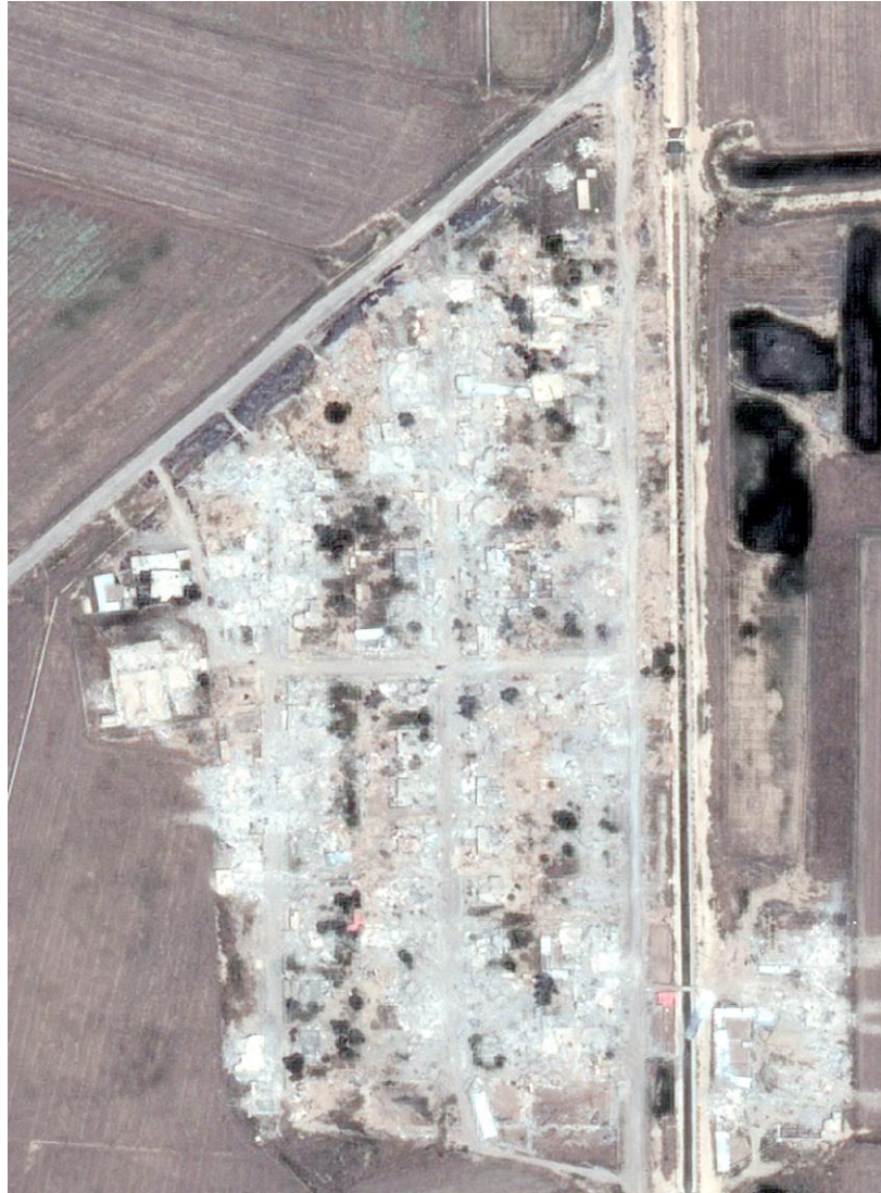
Nahrawan is completely destroyed © CNES 2015
