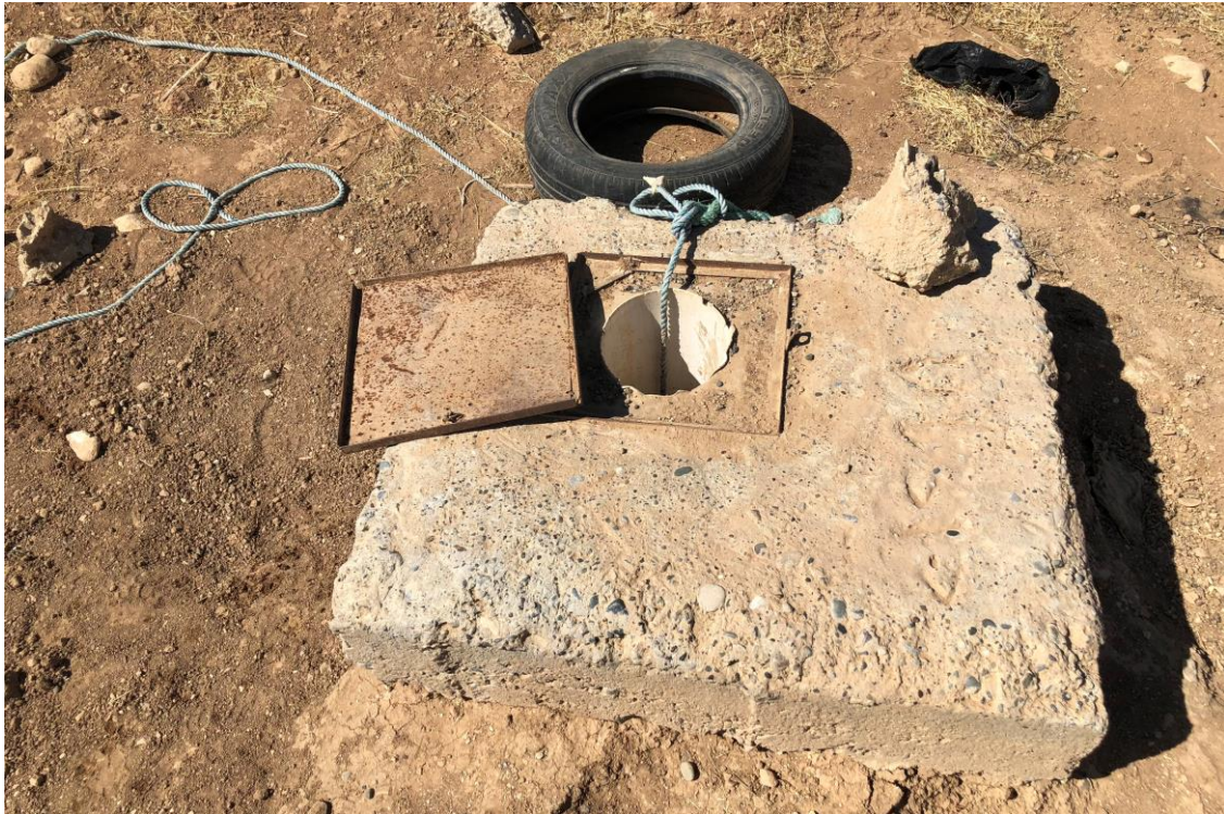
A sabotaged irrigation well on Hakar's farm on the south side of Sinjar mountain. He told Amnesty International: "Without [irrigation] water, I can't grow anything... We cannot afford to fix this, or anything close. © Richard Pearshouse/Amnesty International
