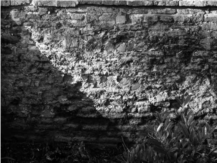
Fig 1.5 Remnant of mediaeval Charterhouse wall
